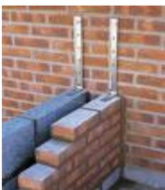
In addition to building this wall from a foundation or lintel, it will also be necessary to tie it into the existing brickwork either side of the opening. This can be achieved by using a proprietary wall starter system (as shown) or stainless steel screw in wall ties. These should be connected to the existing wall, centrally to the proposed brick/ blockwork and tied in at 450 centers.
