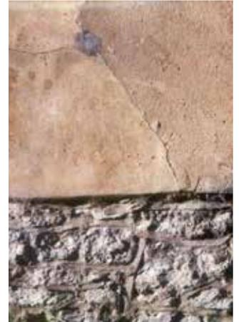
*Cement mortar pointed grumplings and cement render. Cracks in both are drawing in water through capillary action. The moisture is unable to escape through dense render and cement mortar*
