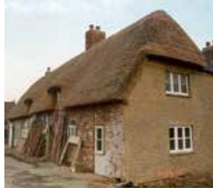
*After repairs with new traditional long-straw roof*
