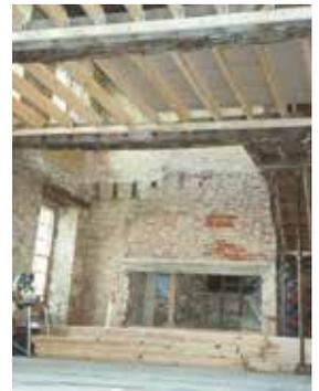
*Damaged listed interior after unauthorised removal of partition walls, joists, floor boards, wall plaster and fireplace surround*
