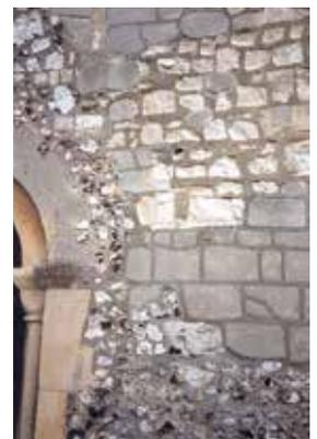
*Inappropriate cement mortar repointing has damaged the soft limestone irreversibly*
