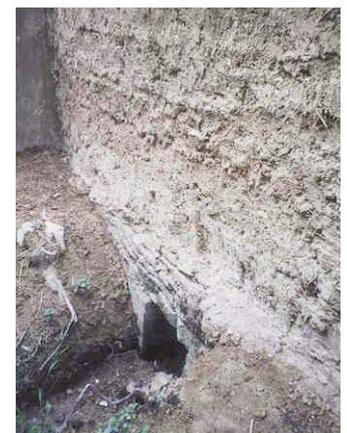
*Newly rebuilt witchert wall over stream before trimming.*
