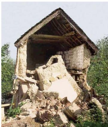
*The photograph shows what happens when the solid ground on which the earth walls are founded, is dug away from below its foundations in order to underpin it. Witchert is a monolithic building material, which cannot cope with the stresses imposed by such massive intervention.*
