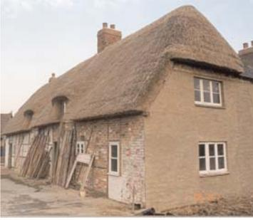
*After repairs with new traditional long-straw roof*
