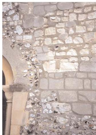
*Inappropriate cement mortar repointing has damaged the soft limestone irreversibly*
